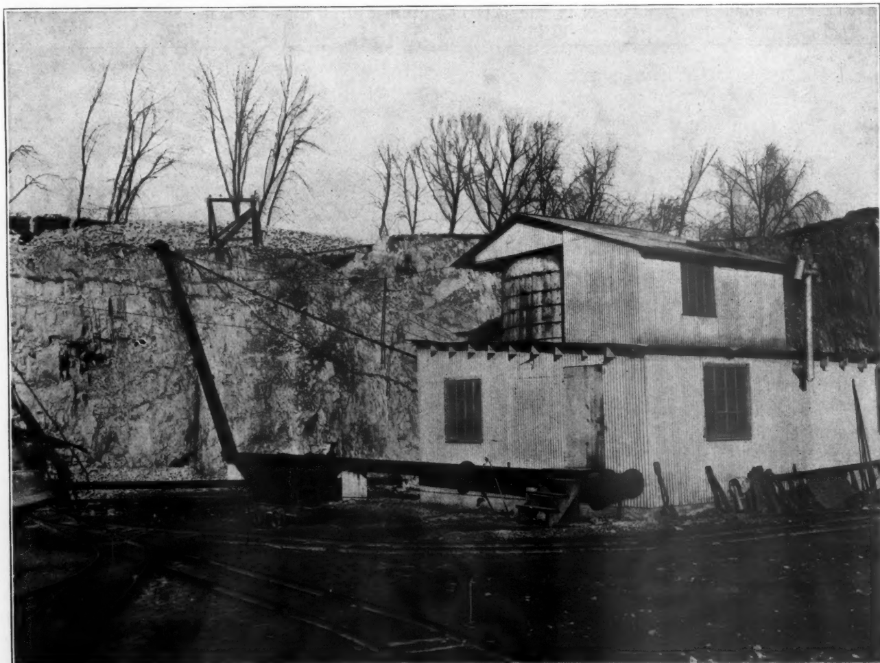
Well House and Suction Pipe at Bottom of Quarry
